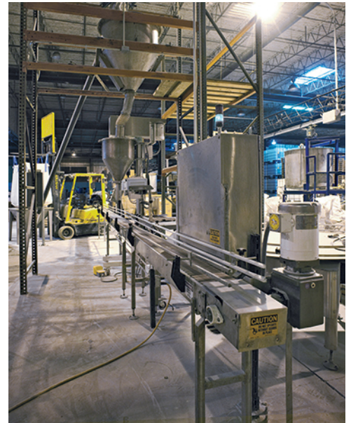
A flexible screw conveyor proved the best way to move the perlite mixture to a ceiling-high surge hopper above the packaging machine.
