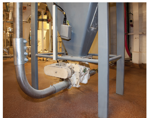
Sugar flows from the floor hopper through a rotary valve into 200 m long PNEUMATI-CON® pneumatic conveying line powered by the blower above the hopper.
