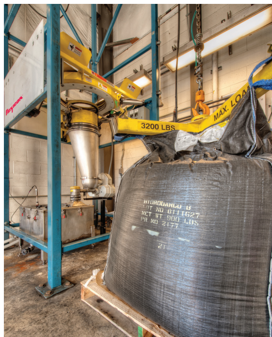
After the lifting frame and bulk bag are fastened, an electric hoist and trolley suspended from a cantilevered I-beam lift and position the bag in the discharger frame.
