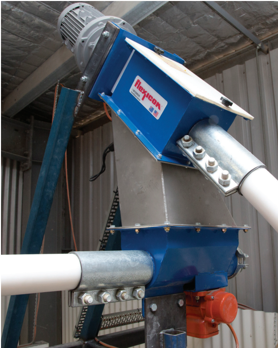
Gypsum powder moves from the bulk bag discharger through the inclined flexible screw conveyor which transitions to a horizontal flexible screw conveyor discharging into the red pelletizer.
