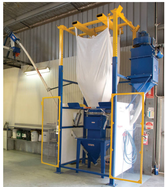
An inclined and a horizontal flexible screw conveyor transport gypsum powder from the bulk bag discharger to the rotary treater.
