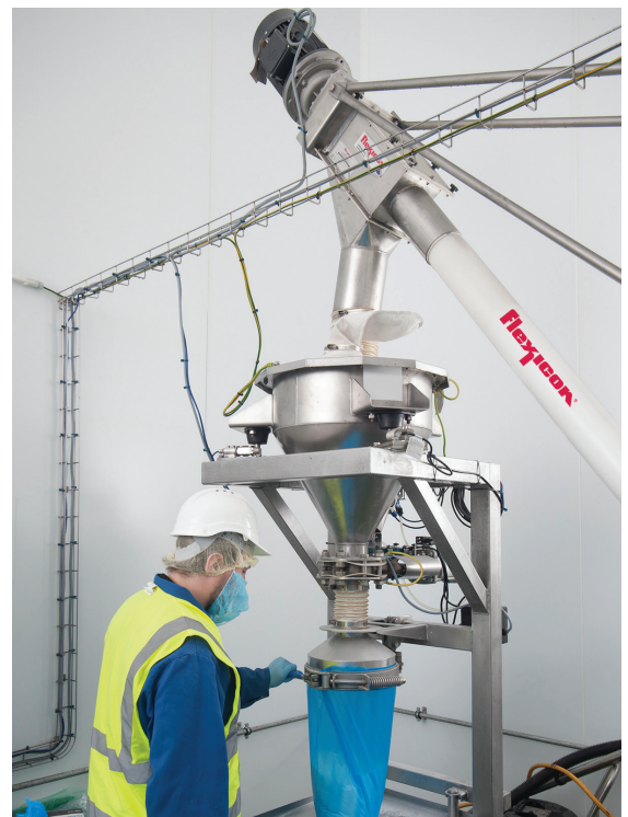
The system controller starts, slows and stops the flexible screw conveyor according to the amount of sugar gained by the gain-in-weight receiving hopper suspended on load cells.
