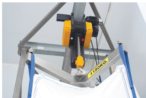
Electric hoist raises the lifting frame and bulk bag, which are rolled into position by a trolley.
