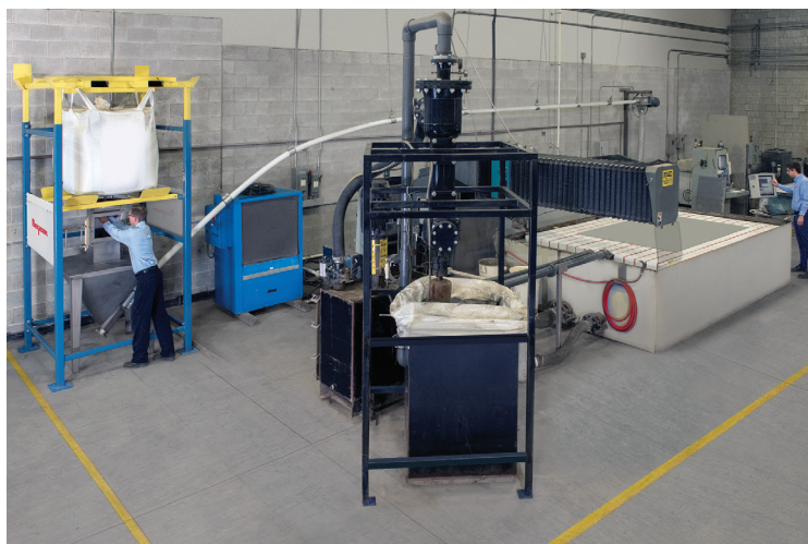
JET-FEED™ garnet delivery system (along back wall) and spent garnet reclamation system (foreground).
