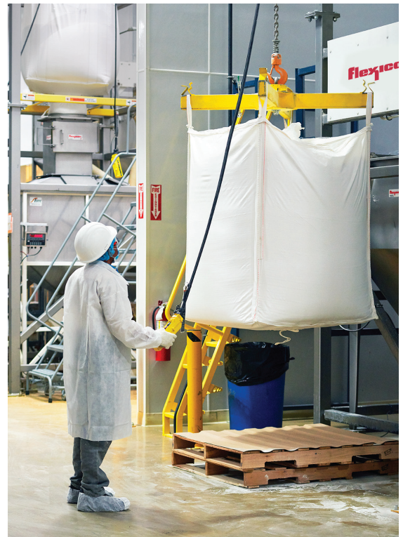
A cantilevered I-beam with hoist and trolley allows bags to be raised and rolled into the discharger using a pendant.
