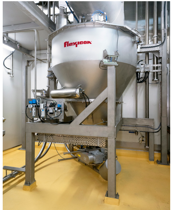
Batches gravity discharged from a mixer into this buffer hopper are conveyed pneumatically to a downstream process.
