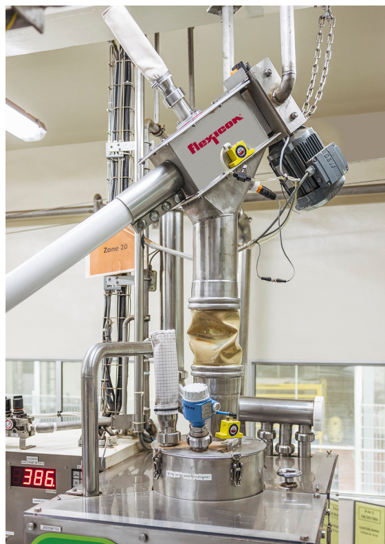
At floor level, an operator attaches bulk bag straps to Z-Clip™ strap holders of a bag lifting frame held in position by a forklift.
