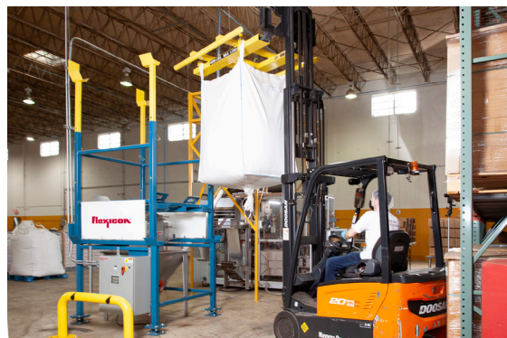
A forklift loads the lifting cradle with suspended bulk bag onto the discharger's receiving cups.
