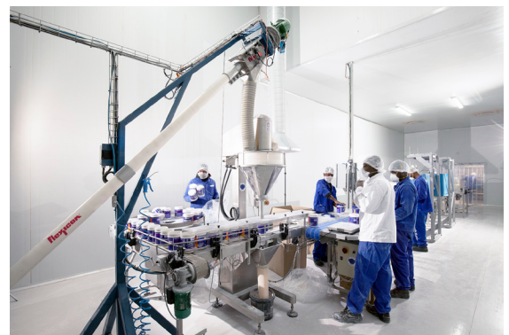
From the discharger's floor hopper, the flexible screw conveyor transfers mixed ingredients to the packaging machine hopper and packaging line. Material remains fully enclosed, preventing contamination.
