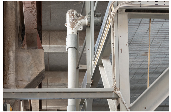
Replacing a failed pneumatic pipe elbow, the HammerTek elbow minimizes wear of the elbow wall as the spherical chamber gently deflects the incoming material around the bend.
