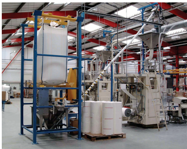
Bulk bag discharger in foreground delivers silica gel granules through receiving hopper and flexible screw conveyor, at 45°, to the first of four feed hoppers.
