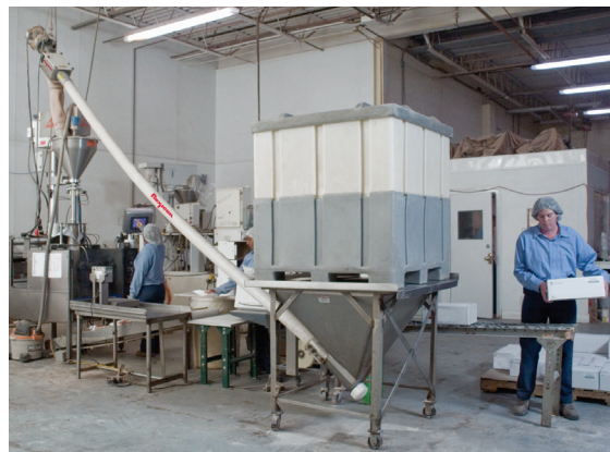
Each flexible screw conveyor transports powder at a rate of 140 cu ft (42.7 cu m) per hour 12 ft (3.7 m) above the plant floor for discharge into each packaging machine.
