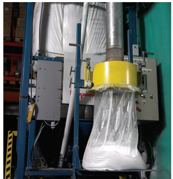
When the weigh hopper reaches its target weight, the batch of clay is discharged into a bag and taken to the blender.
