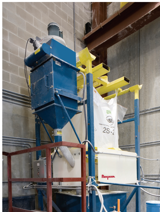
Two bulk bag unloaders unload and transfer 4000-6000 lb (1814-2722 kg) per day of diatomaceous earth (DE) for Tampa Bay desalination plant's DE filtration system. The crane deposits a lifting frame holding the bulk bag onto the unloader frame.
