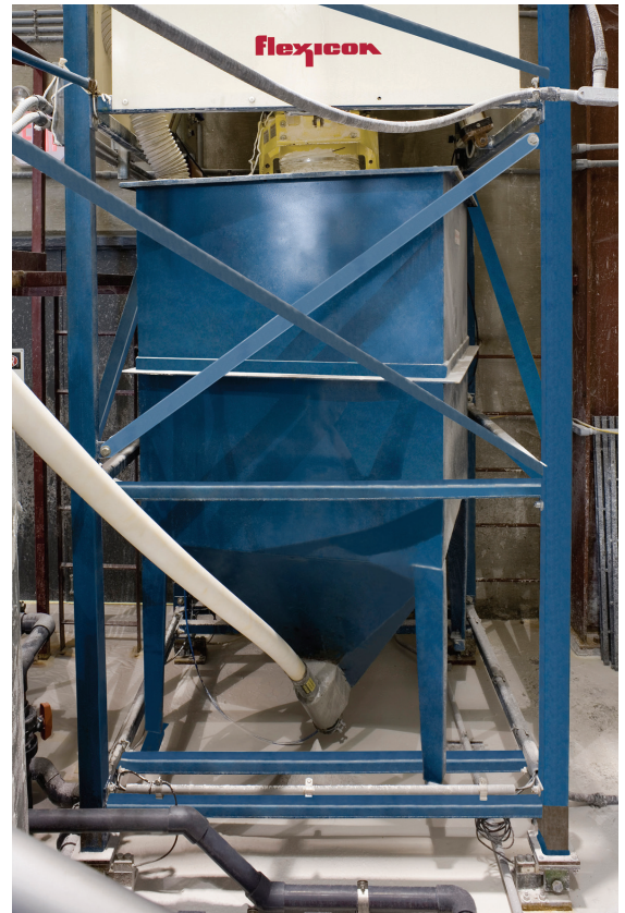
The 63 cu ft (1.8 cu m) capacity hopper holds the contents of a 900 lb (408 kg) bulk bag allowing diatomaceous earth to transfer, unattended, through the flexible screw conveyor to the tank. Load cells under the unloader frame transmit weight loss information to a PLC to achieve accurate batch weight transfer.
