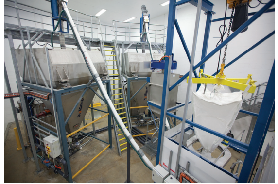
Two flexible screw conveyors feed fluoride powder from the bulk bag discharger into two seven-day storage hoppers from which the powder is metered into two mixing tanks for dosing into the main water supply.
