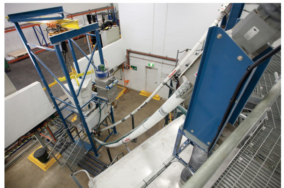
Two flexible screw conveyors feed fluoride powder from the bulk bag discharger into two seven-day storage hoppers from which the powder is metered into two mixing tanks for dosing into the main water supply.
