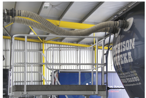
One pneumatic line discharges into the tanker's inlet port, while a second line vents an outlet port, leading to a filter receiver where dust is separated from clean air vented to the atmosphere.
