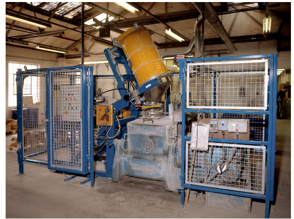
At the drum discharge station, a cone seats against the drum rim and the receiving hopper inlet, preventing dust as dry material is transferred to the wet blender.
