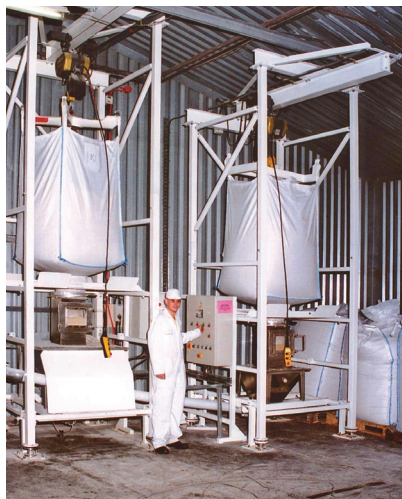
Flexicon (Europe) Ltd. designed and installed two Bulk Discharge Handling Systems at cookie maker Simmens of Edinburgh Ltd. One is for medium-grain oatmeal (left), the other for fine-grain oatmeal.
