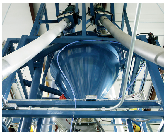
Flexible screw conveyors slow to dribble speed for pinpoint accuracy in measurement of ingredients to within 1% of recipe targets, and also isolate the powders from moisture in plant air.
