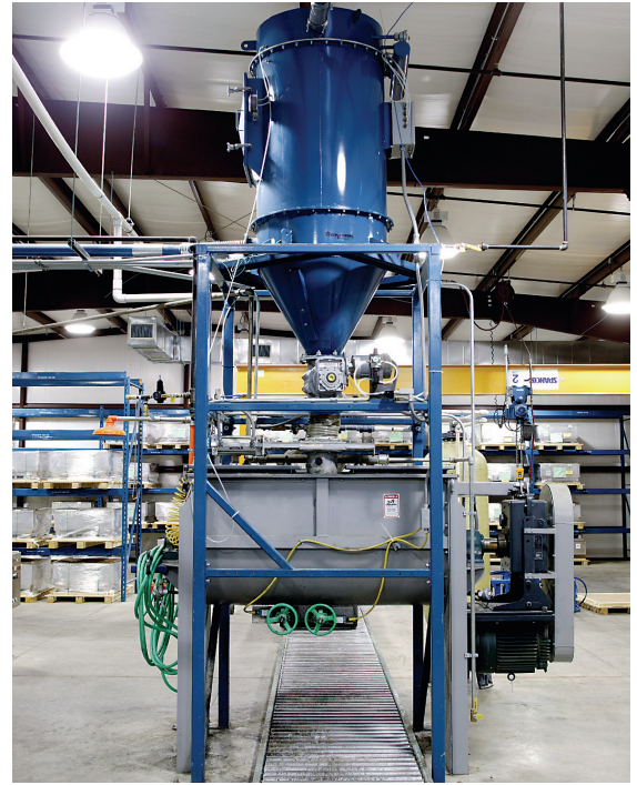
A filter-receiver with reverse-pulse filter cleaning continuously and efficiently separates the powder from the vacuum pneumatic system, dropping process feed into the wet mixer.
